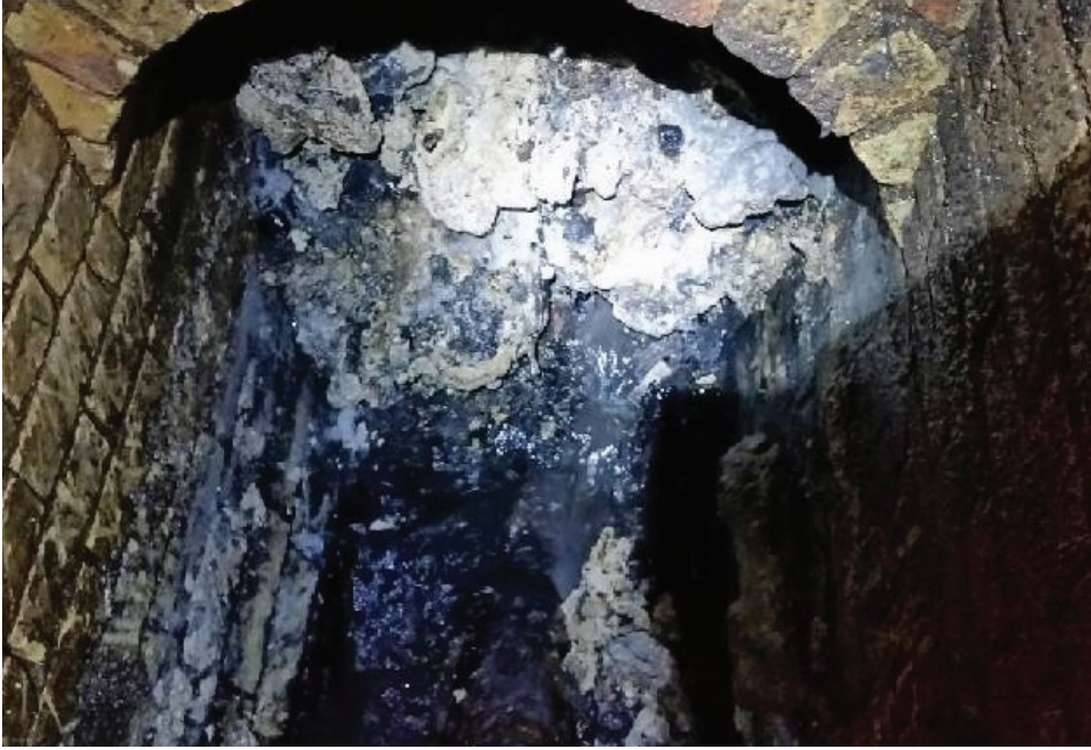
A world famous fatberg clogging the Victorian sewers of Whitechapel, London in 2017. This photo by Thames Water contributed to its fame. Photo: Thames Water.
