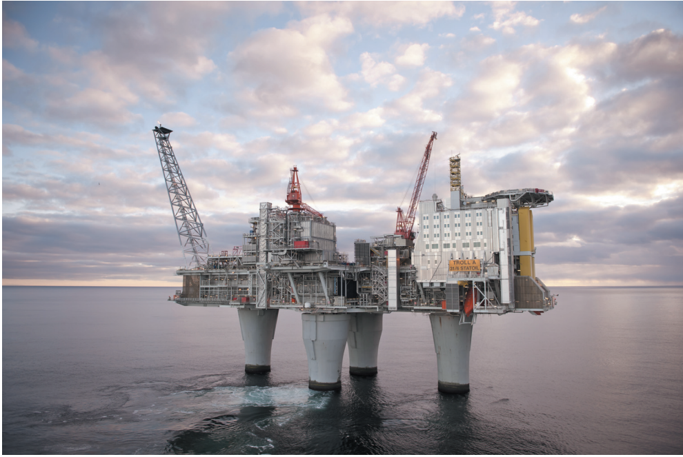
Gas-producing Troll. A platform on the Troll field. Photo: Øyvind Hagen, Equinor.
