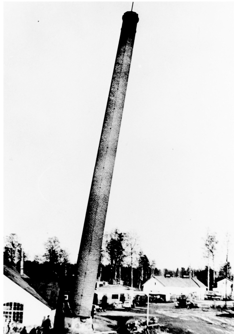
Demolishing the smokestack in 1966. Photo: The Archive of Traditional Society of Ähtäri.
